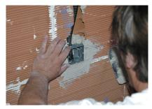
13. Another option is to execute the finish using drywall panels .It is very important that the juncture boxes protrude about 15mm because they have to be levelled when the drywall panel is fixed.
