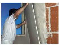
15. The plaster must be uniformly spread, it is essential to achieve a perfect fixation of the drywall panel (from the floor to the ceiling).
