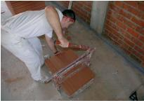
**6.** The large- sized brick HispaPlano is easily cut using the guillotine even for an inexperienced person. The cut is accurate, easy and fast.
