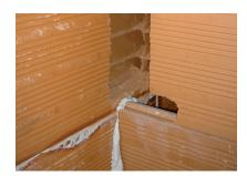
**8.** The interlockings for junctures to partitions must be done in the even numbered course (2<sup>nd</sup> and 4<sup>th</sup>). The quality of bricks HispaPlano allows to make interlocks easily, the pieces are perfectly fitted keeping their integrity.
