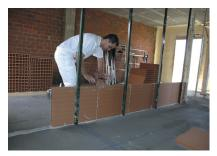
**4.** Before laying the first course of clay large – sized bricks, it is necessary to put mortar on the perimeter tape to fix the partition.
