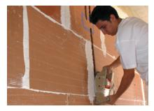
11. Thanks to the quality of the bicks HispaPlano, the channels for electric and plumbing installations and also the spaces for the juncture boxes can be easily executed using a radial tool.
