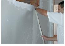
18. The joints among the panels must be filled using plaster. The tape is placed on the plaster to avoid crack forming. This tape is fixed using a second application of plaster.
