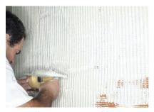
14. Equidistant masses of fixing plaster Hispalam must be applied on the ceramic partition HispaPlano and then one has to spread them uniformly on the whole surface using a serrated trowel, the resulting layer will not be more than 1cm thick.
