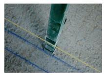
2. The screeds must be carefully fastened and aligned with a string. The suitable distance between two screeds is 70cm approximately.
