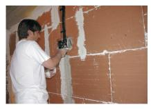
12. After the installation of pipes, boxes and installations, the 100% flatness and the rate water absorption ( $\leq$  10 %) allow a perfect finish using wet plaster (6-15mm).
