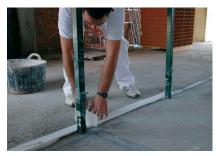
**3.** It is necessary to place elastic perimeter tapes along the layout to insulate the partition from other structural elements.
