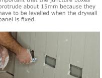
16. After that, it is necessary to mark and open the spaces for juncture boxes.
