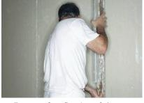
17. For a perfect fixation of the drywall panel to the ceramic partition it is essential to use a screed. In this way, the joints of the partition Hispalam are ready for being covered using a tape.
