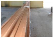
**5.** The clay large- sized bricks are tongued and grooved so they are accurately fitted. Mortar is applied on both sides of the tongued edge to get secure fixation to the upper course.
