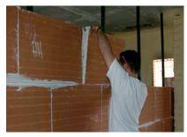
7. The laying of pieces must be staggered; the vertical joints must never coincide.
