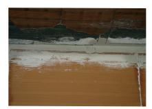
**10.** The juncture to the upper floor structure is executed leaving a joint of 3 or 4cm that will be filled with controlled – set plaster.
